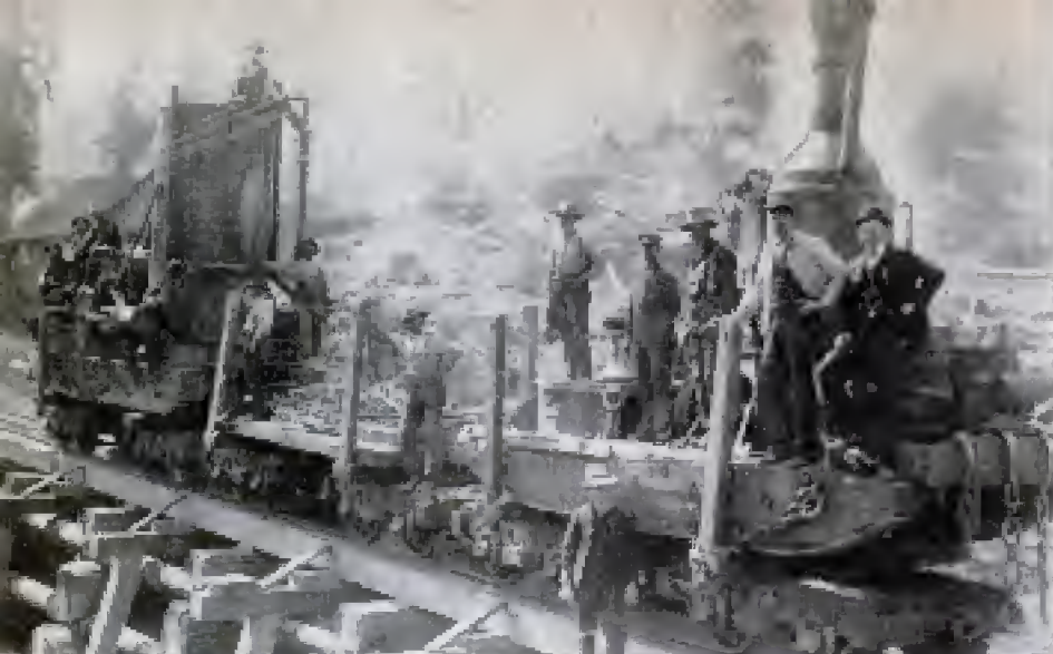
This was a big moment—the arrival of two new “donkeys.” Their cables were snagged around stumps and the donkeys pulled themselves off cars
